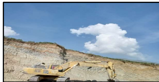
Gambar 4 Excavator Komatsu PC 400
